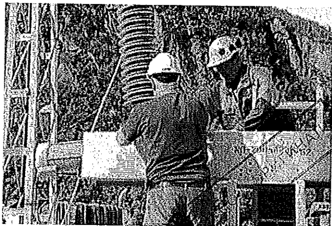
Disconnecting circuit breaker LTB DCB for 145 kV with the operating mechanism Motor Drive installed at refurbishment in Norway.
